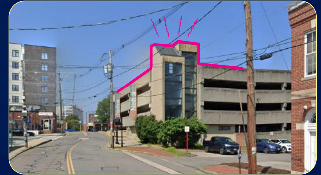
C. View from Main Street to High Street Garage
