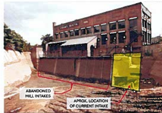
Figure 7-1: Photo of old mill intake dewatered prior to the installation of the existing intake
