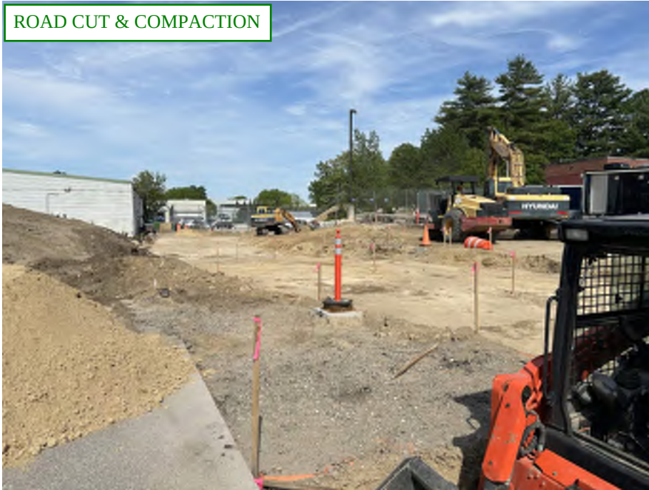
ROAD CUT & COMPACTION, DEMO'D LIGHT POLES & ISLANDS
