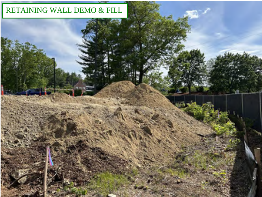
RETAINING WALL DEMO & FILL
