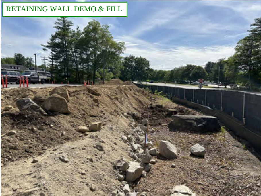
RETAINING WALL DEMO & FILL
