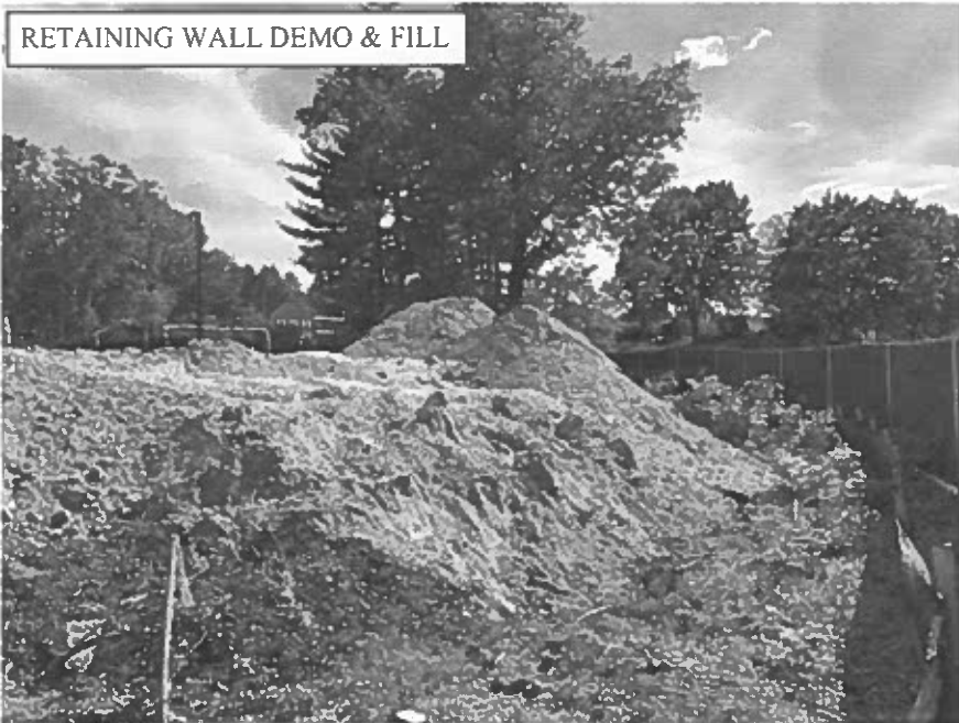
RETAINING WALL DEMO & FILL
