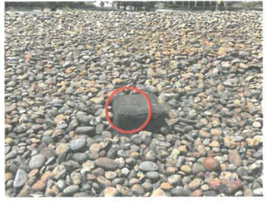
8. Multiple holes in found in flashing of obsolete penetration. Provide new EPDM flashing in accordance with Carlisle guidelines.
