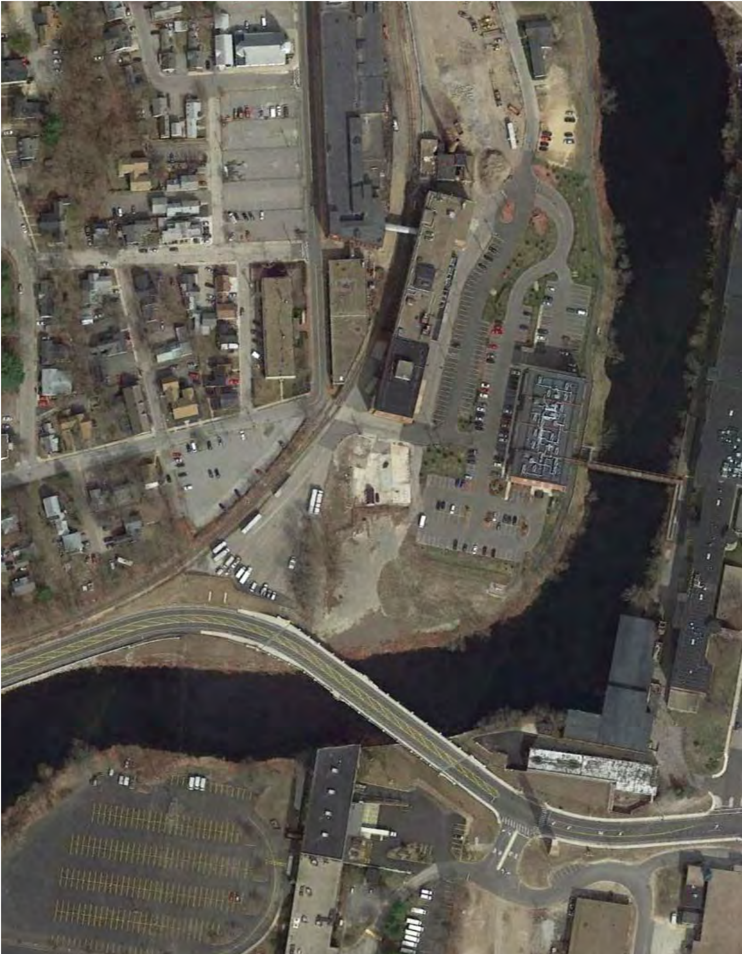
Aerial of Existing Conditions at Greeley & Cotton - West Focus Area
